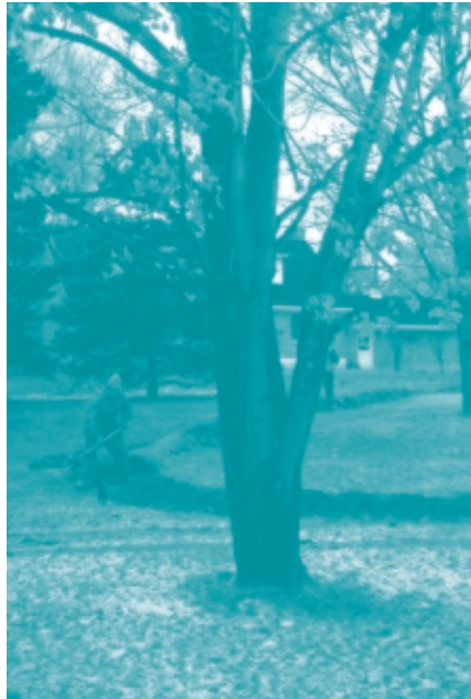
Installation of a ground loop for an existing home.
