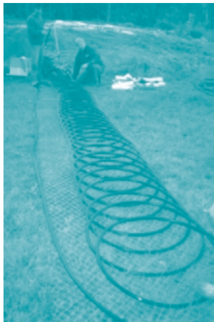
A coiled loop can be installed in the ground or in a pond or lake.
