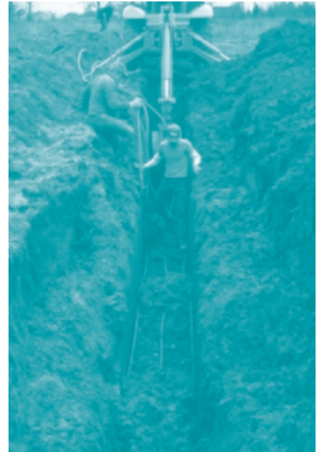
A backhoe is used to dig a horizontal trench for laying a ground loop.
