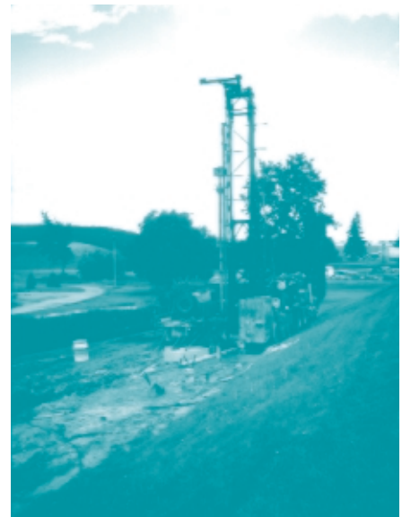
A drilling rig is used to install vertical boreholes.
